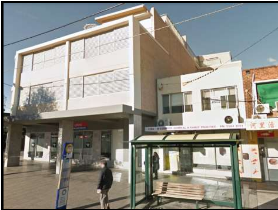
Photo 3: Recent development at 260 Belmore Road Riverwood
