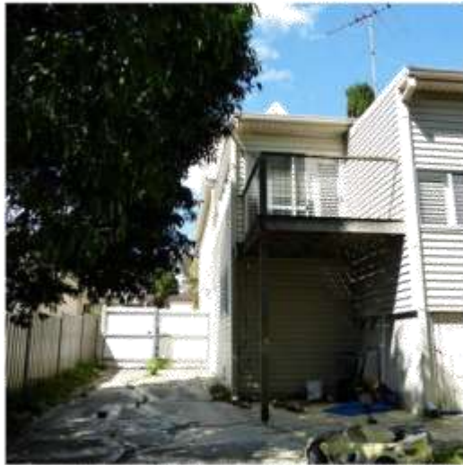
Figure 4.10 | View of western rear of house from back garden. The block slopes down from the road. Gates will partially conceal new carport from street view. The driveway will be removed and replaced during works, due to its damaged state.
