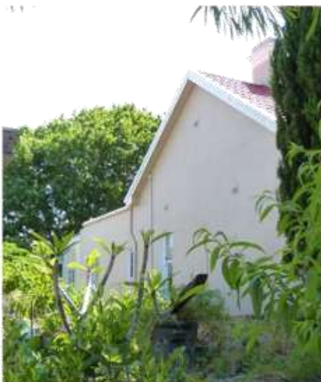
Figure 4.3 | Eastern side of the property, showing the main gable and the skillion roof behind parapet wall over the rear wing of original house. Addition evident at far rear.
