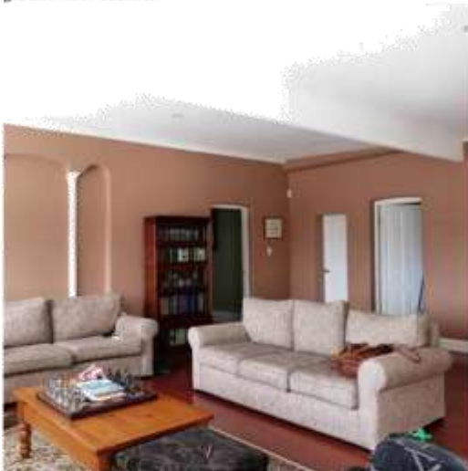
Figure 4.13 | Rear wing of original house. The internalized parapet wall molding seen at ceiling level. Middle door is a small bathroom, door at right will be a study. Proposal is to build a hallway from the original rear door (left) past this rear wing into the first floor addition at the eastern rear.
