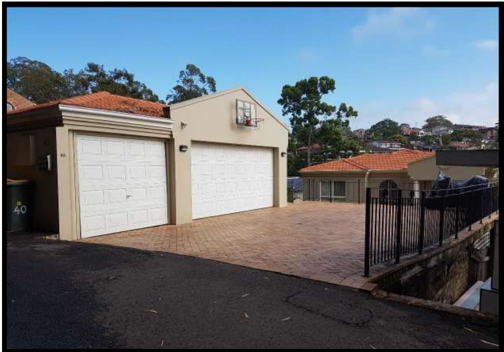
Adjoining property to the west – 40 Herbert Street Oatley
