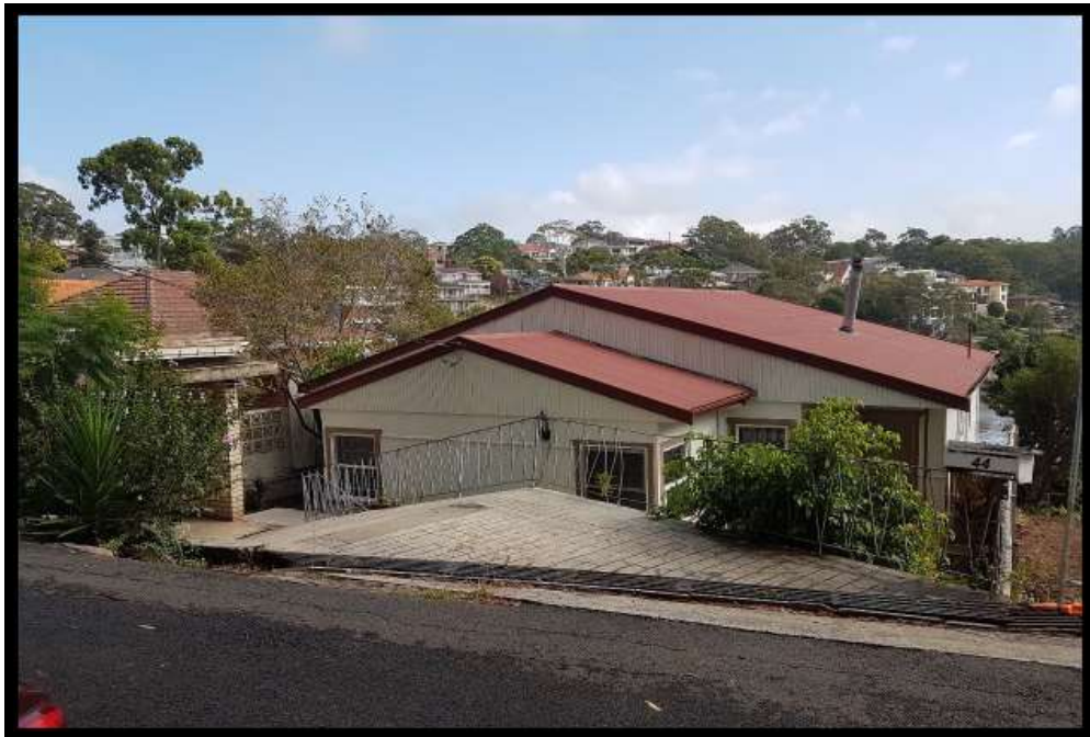
Adjoining property to the east – 44 Herbert Street Oatley
