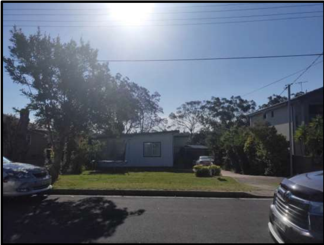
Figure 5: Photograph of subject site - western aspect (57-59 Clarke Street, Peakhurst) viewed from Clarke Street (Source: GRC, 2019)
