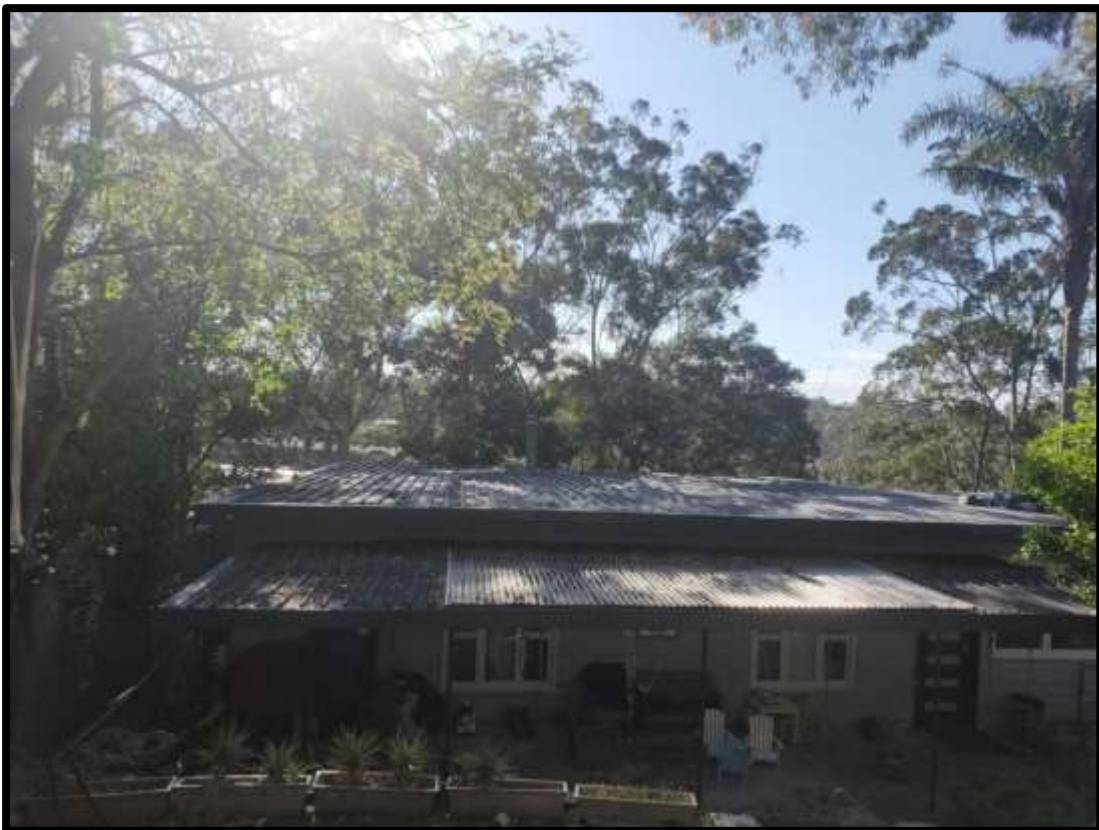
Figure 6: Photograph of rear of subject site (57-59 Clarke Street, Peakhurst) along western aspect. (Source: GRC, 2019)
