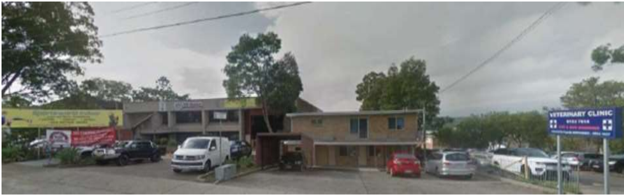
Figure 9 – Commercial development 707 Forest Road, Peakhurst (West)
