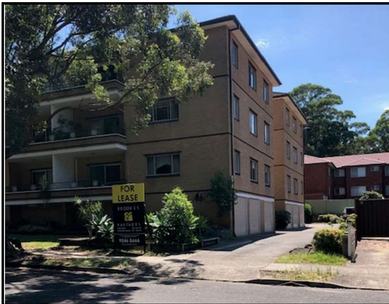
Figure 9: Adjoining development to the north, 50-52 Noble Street Allawah
