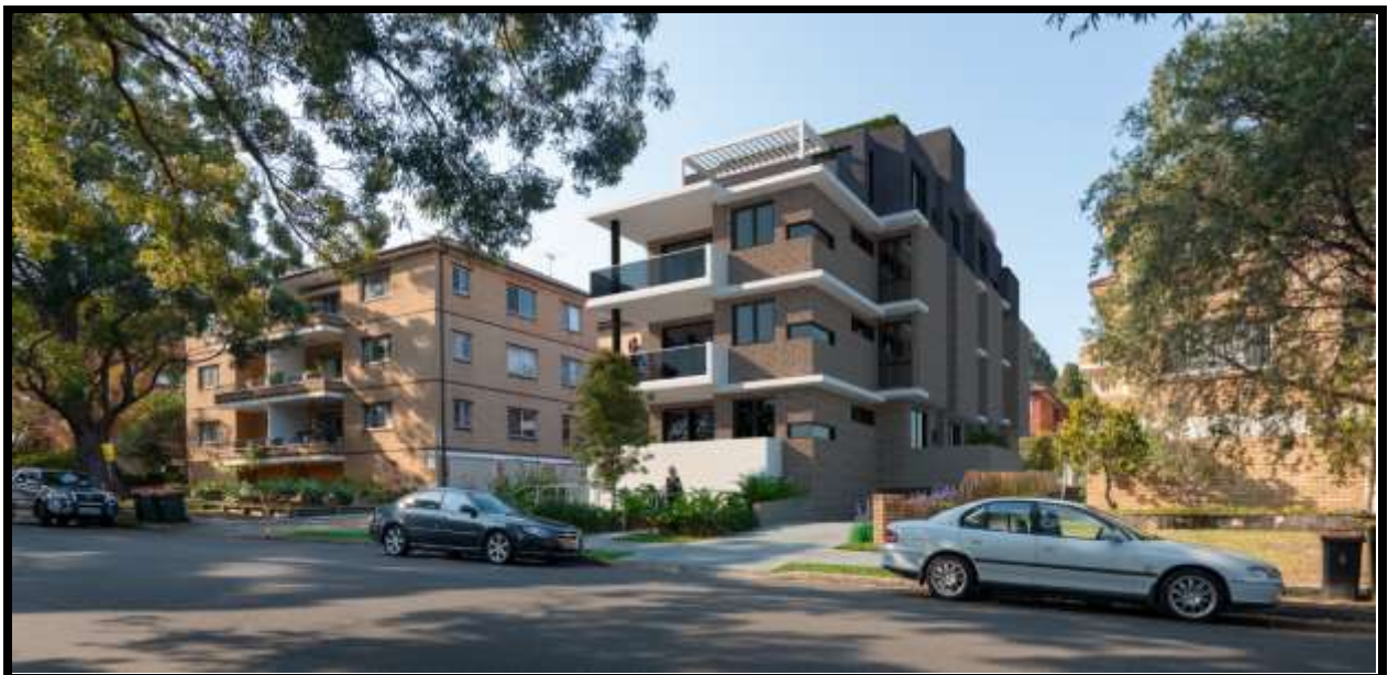
Figure 2: 3D Montage of the amended proposed RFB refused under DA2019/0314 (Courtesy: Cornerstone Design, March 2020, Issue B)
