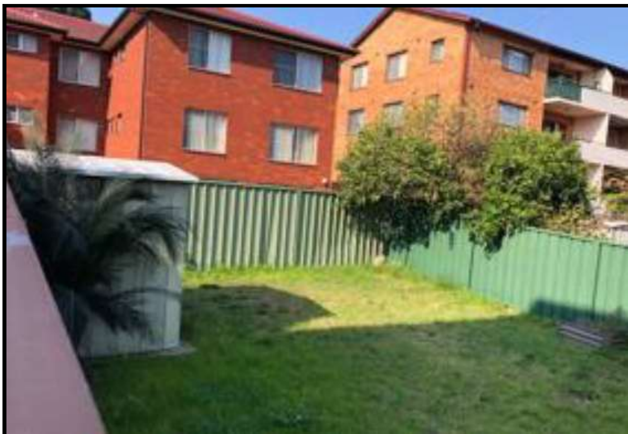
Figure 10: Development at the rear of the subject site, 43 and 47 Illawarra Street.
