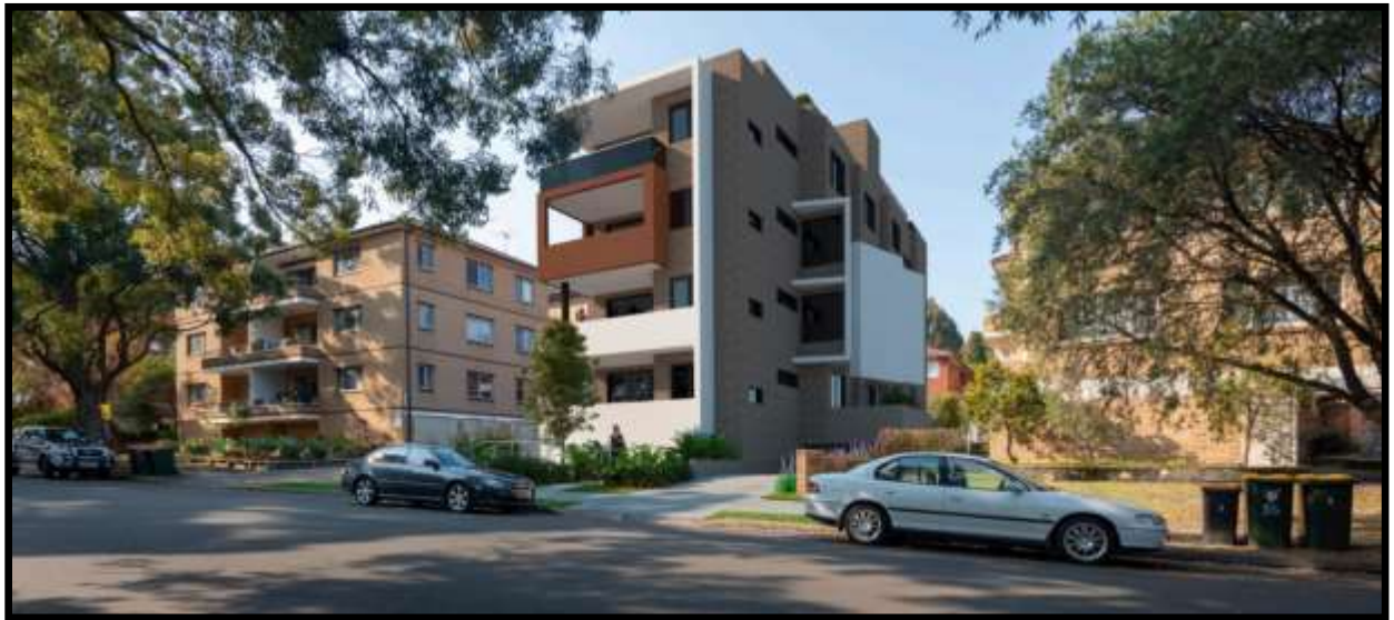
Figure 1: 3D Montage of the originally proposed RFB (Courtesy: Cornerstone Design, June 2019 Issue A)
