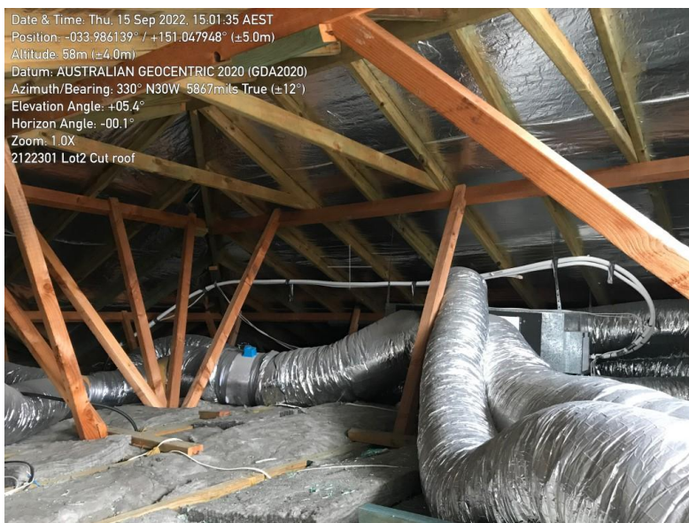
Image 10 – Timber roof framing system.
