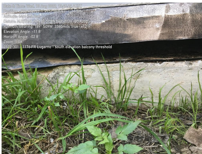
Image 3 – Sheet membrane on balcony slab typical.
