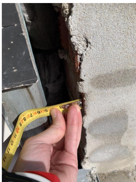
Image 8 – First floor brick veneer wall cavity.
