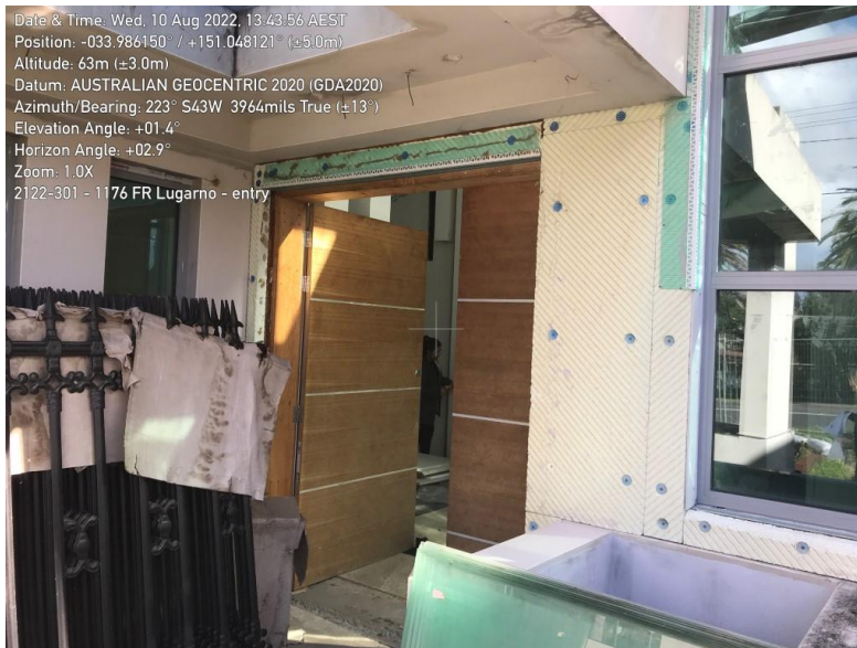
Image 1 – Lightweight wall at entry portal.
