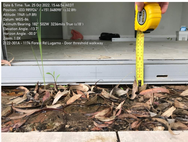
Image 21 – Door threshold external to internal FFL (ground floor).
