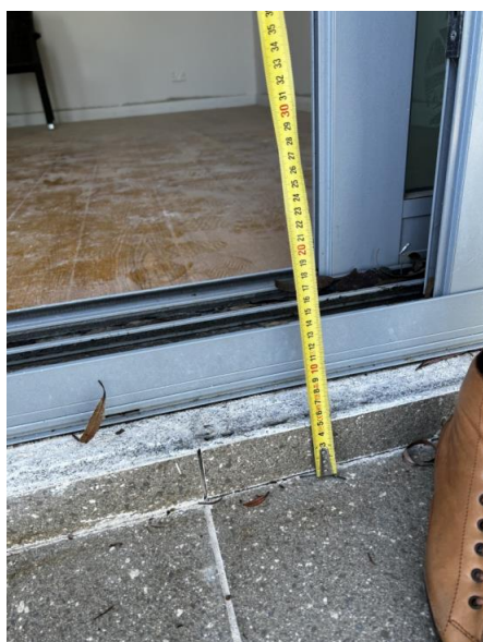
Image 22 – Door threshold external to internal FFL (first floor).
