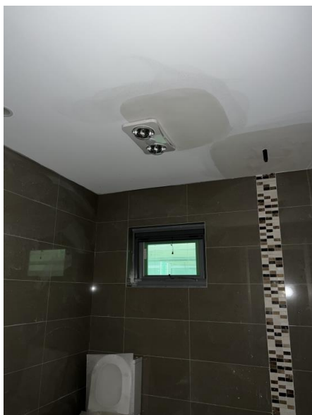
Image 7 – Water damage to bathroom ceiling.
