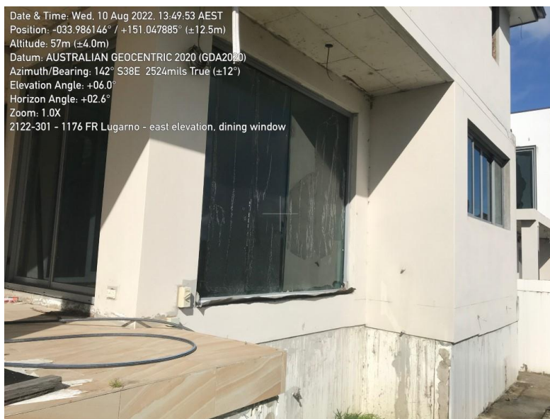
Image 4 – Dining room glazing damage.
