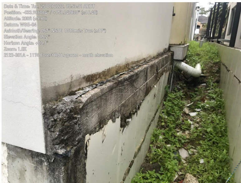
Image 11 – Damp Proof Course to underside of brick wall.
