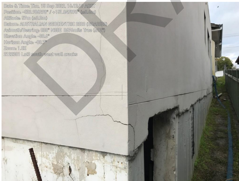
Image 4 – Cracking in render to southwest corner.
