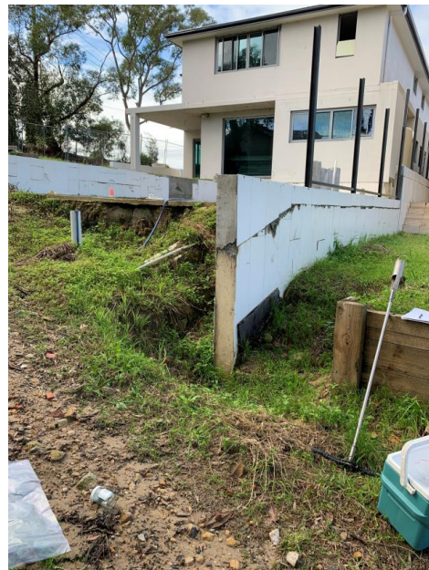
Photograph 10: Western portion of 1174-1176 Forest Road. Image shows exposed fill material including crushed bricks, tiles concrete.
