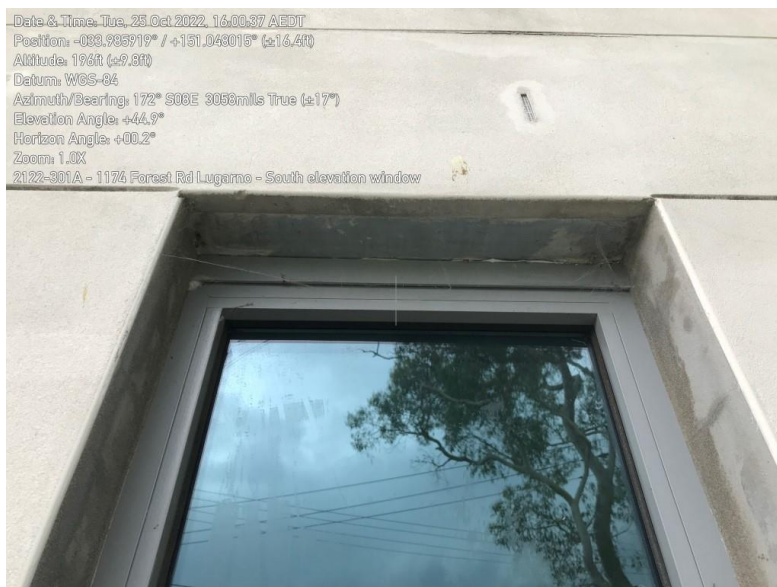
Image 18 – Window with head flashing (typical)
