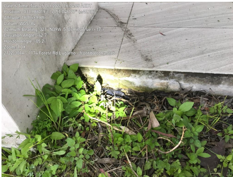
Image 13 – Front balcony slab with pliable membrane underside.
