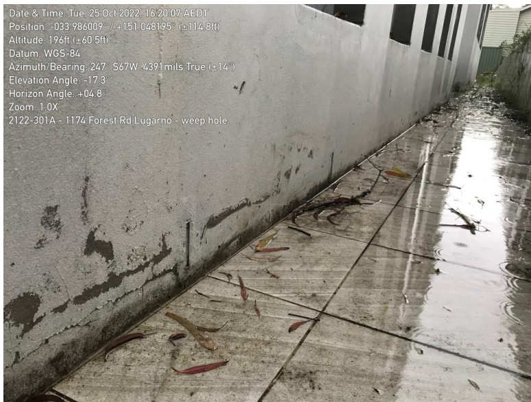
Image 17 – Weepholes installed to bottom of external wall.
