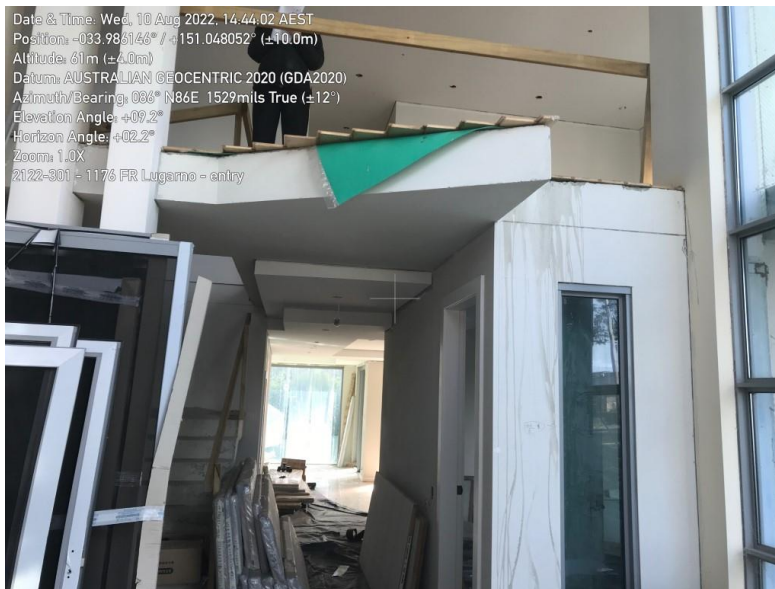
Image 5 – Landing and stairway temporary barrier.
