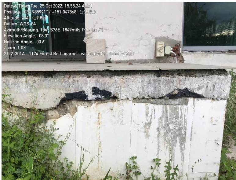
Image 12 – Rear balcony slab with pliable membrane underside.
