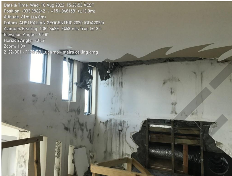
Image 12 – Ceiling damage to the landing.
