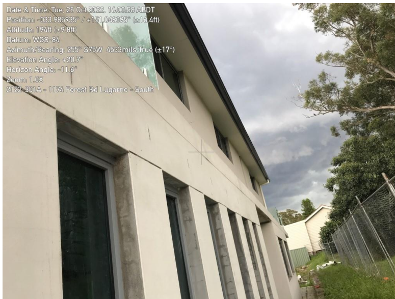
Image 16 – Weepholes installed to interstory junction.
