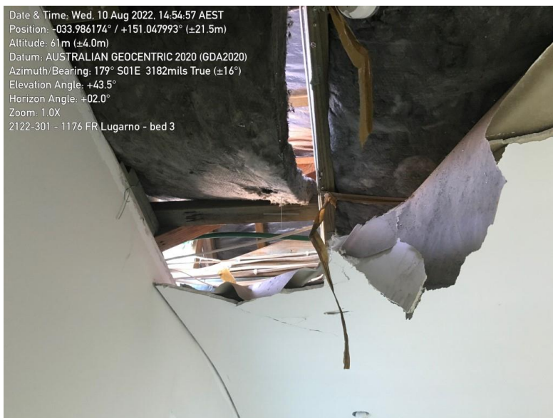
Image 7 – Bedroom 3 ceiling damage.
