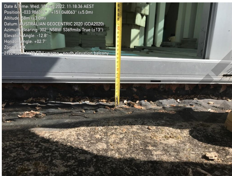
Image 1 – Brick course to FFL upturn height typical.
