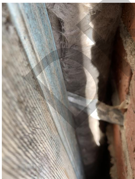
Image 12 & Image 13 – Brick veneer wall insulation & brick ties.
