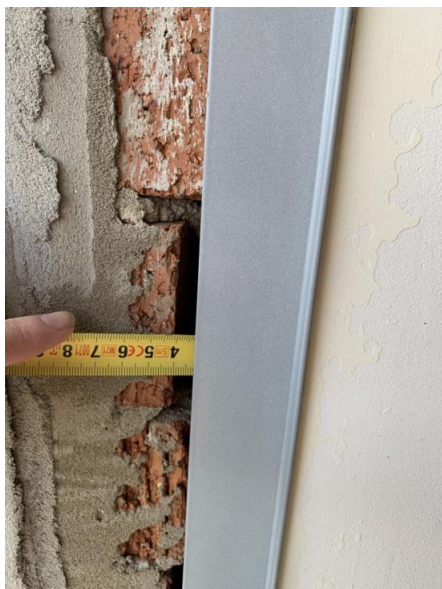
Image 8 – Cavity brick wall cavity width.
