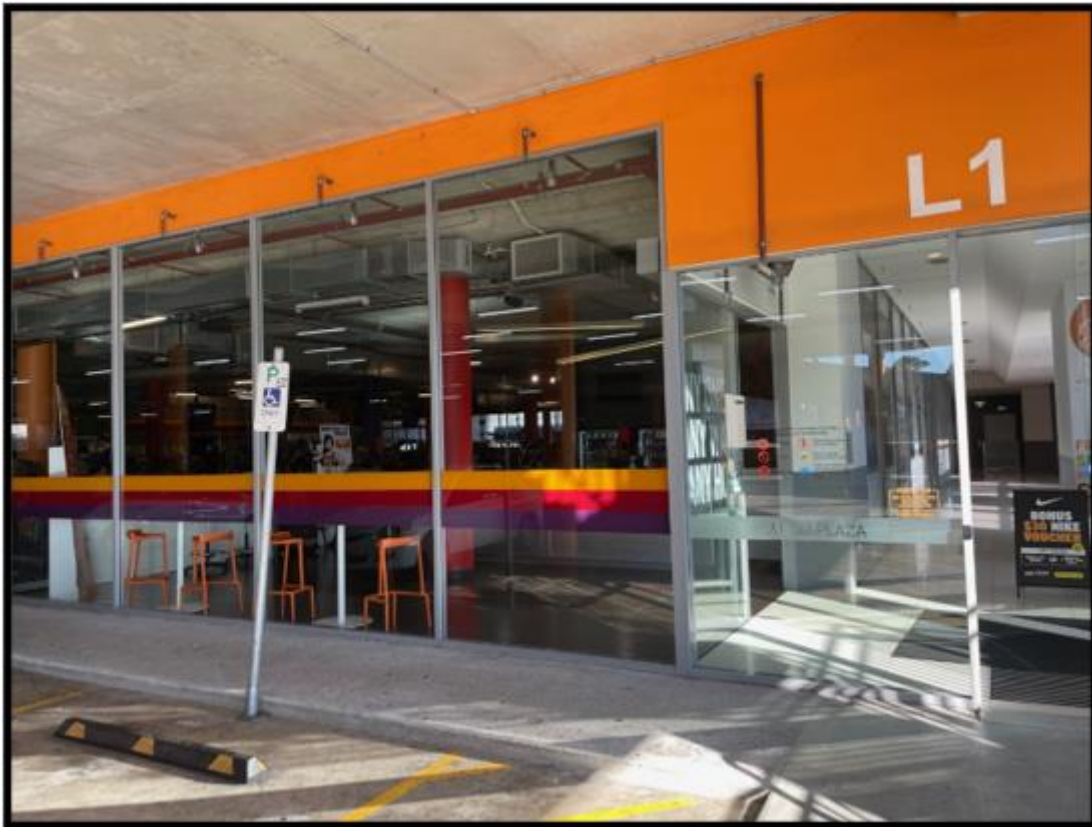
Figure 7: Photo taken within the building from the first floor - 84D Roberts Avenue, Mortdale
