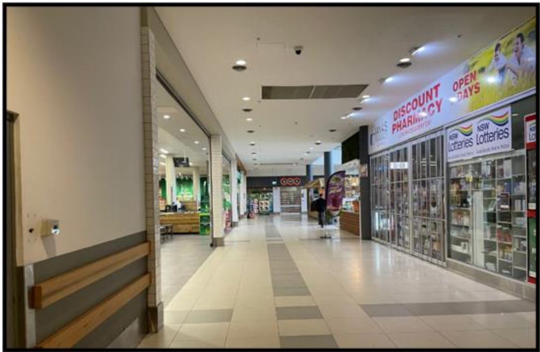
Figure 6: Photo taken within the building from the ground floor - 84D Roberts Avenue, Mortdale
