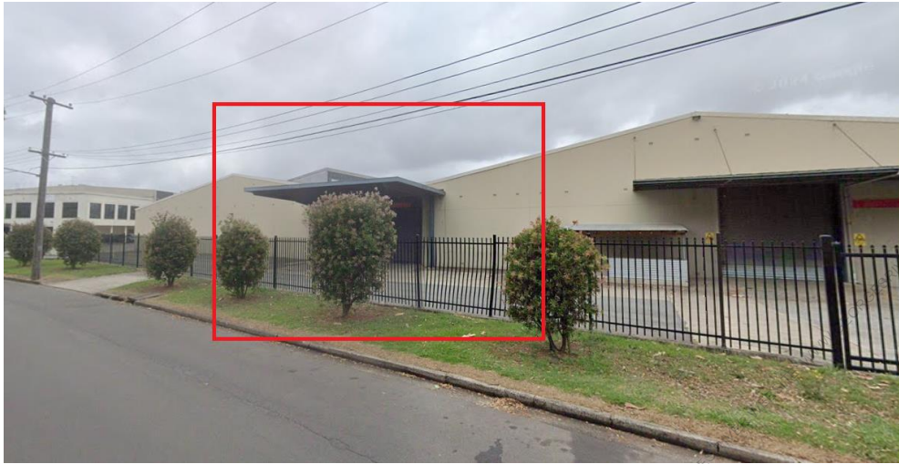
Figure 3: Street View from Crescent Street (Google Maps, 2025)
