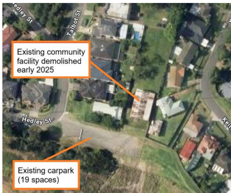
Figure 9: Aerial image showing demolished community centre (Source: Google Maps)
