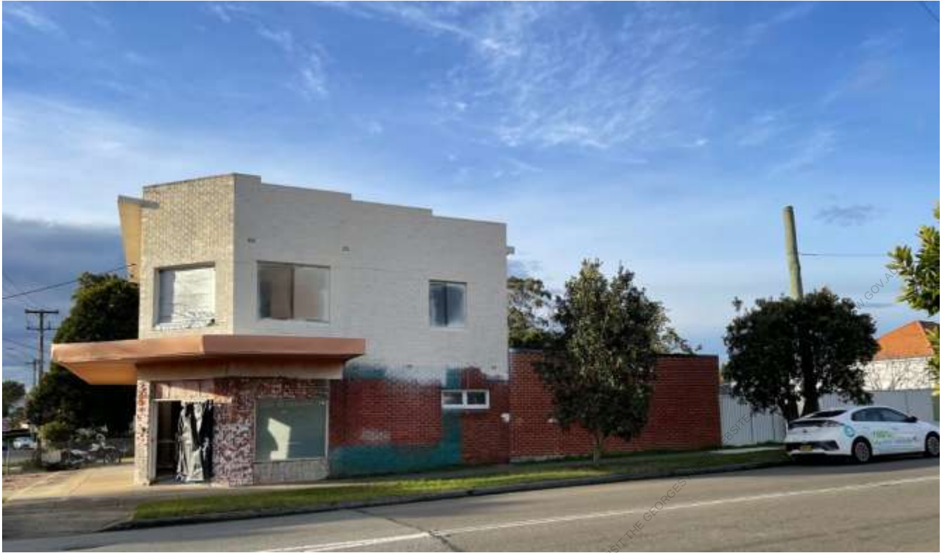
Figure 5: Subject site – Isaac Street frontage.
