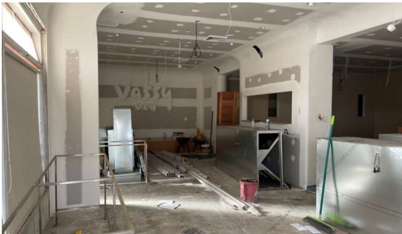
Figure 7: Subject site – Internal works.
