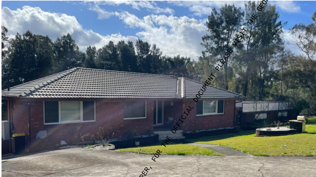
Figure 8: Street view of development site (Image taken facing South/East/West/North (Source: Assessing Officer))
