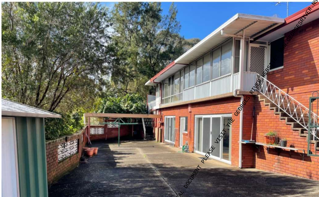
Figure 7 – View of the existing private open space (Source: Assessing Officer)
