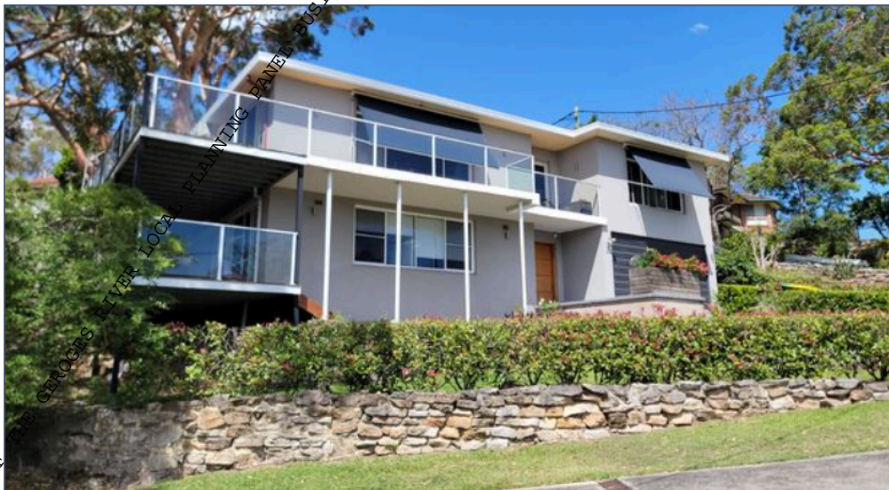
Figure 12 – Front facing windows and balconies at 1 Dinjerra Crescent (Milou & Associates)
