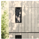
5 CONCRETE PANEL RAW OR WITH IVORY RENDER FINISH IF REQUIRED
