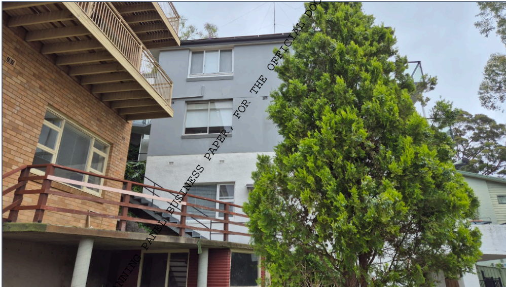
Figure 6: View towards the southern neighbour at 4 Dinjerra Crescent (Corona Projects, 2025)
