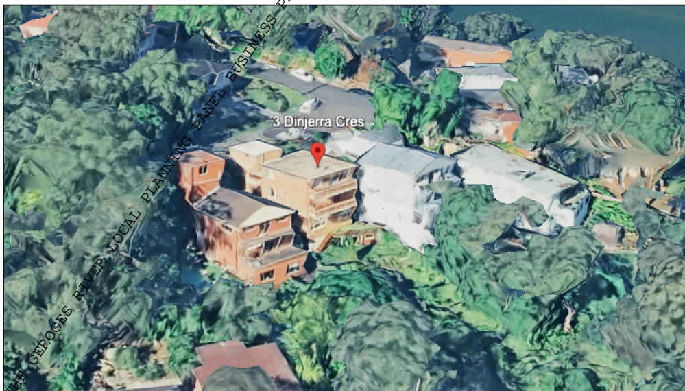
Figure 5: Existing dwelling aerial imagery (Google Earth, 2025)
