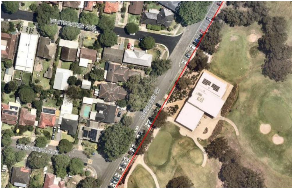
Figure 2 - Aerial of Clubhouse
