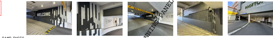
9 ROSE STREET - RAMP PHOTO 1: 100
