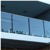
Proposed Glass Balustrade with interlinking Metal Handrail
